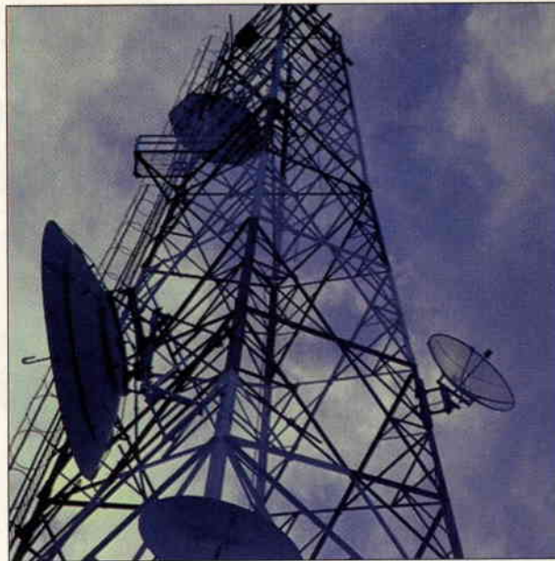
Strides in communications technology continue to revolutionize construction methodology. The Internet will make up-to-the-minute information available to an unlimited number of users.
